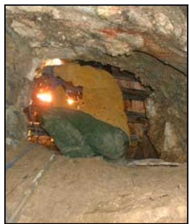
Installing the cave gate at the Timpanogos Cave exit. NPS Photo.
