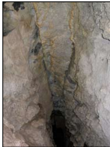
The Middle Cave fault line. NPS Photo.
