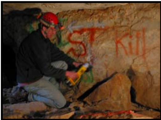
Angle grinding off graffiti Jon Jasper
