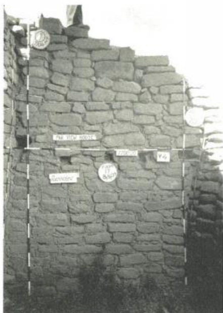
This 1934 photo shows wall sockets and stonework extending well above the sockets, indicators that this part of the ancient structure was at least 2 stories tall.
